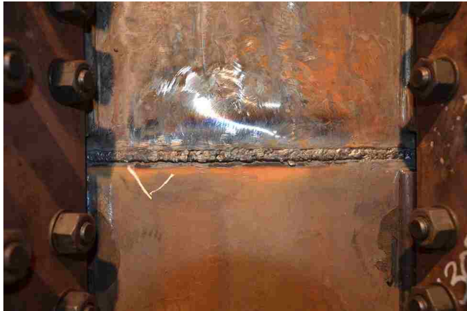
Figure 114 Weld root after removing of backing bar
