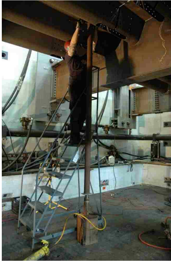
Figure 110 Jacking of west panel
