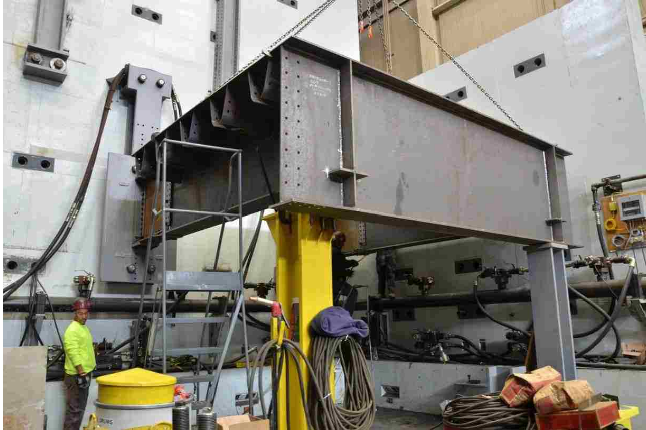
Figure 105 Installation of the east panel
