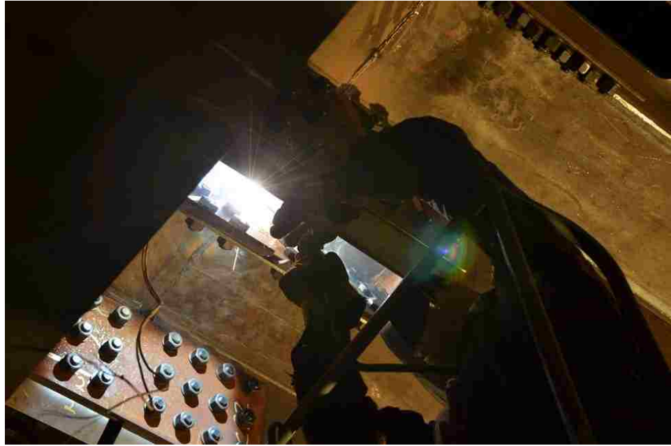
Figure 116 Extensive efforts for back gouge and re-welding inside the rib
