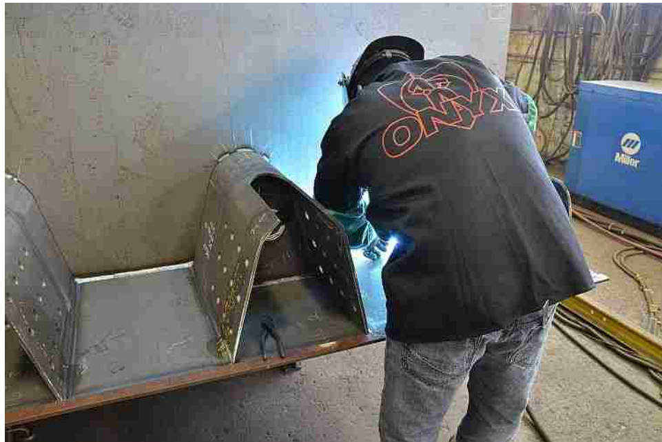
Figure 100 Floor beam-to-deck plate welding
