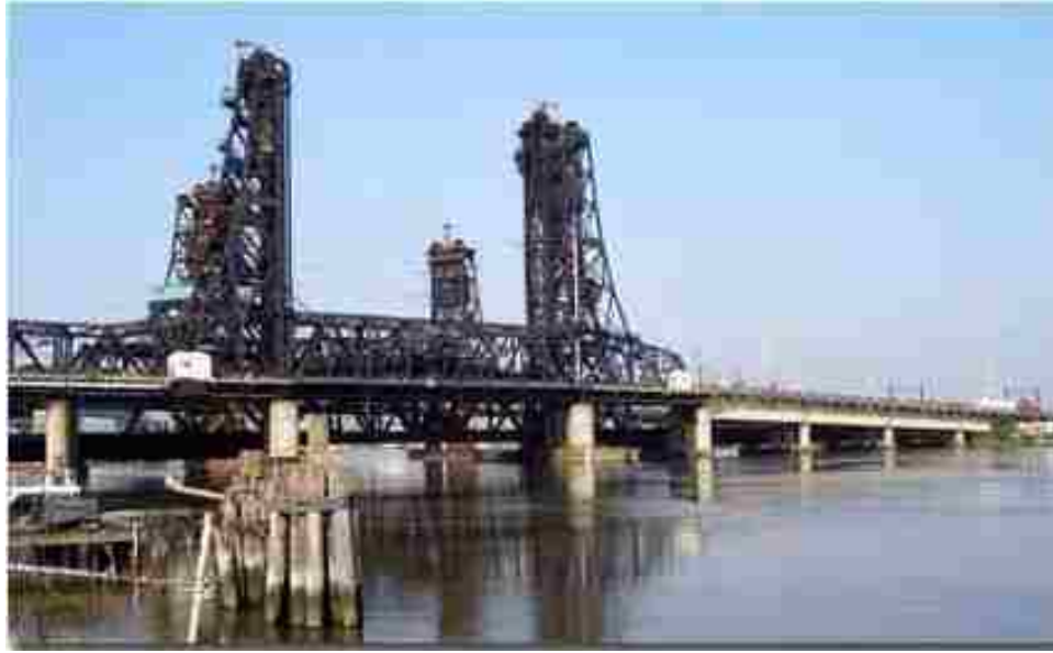
Figure 1 The lift bridge
