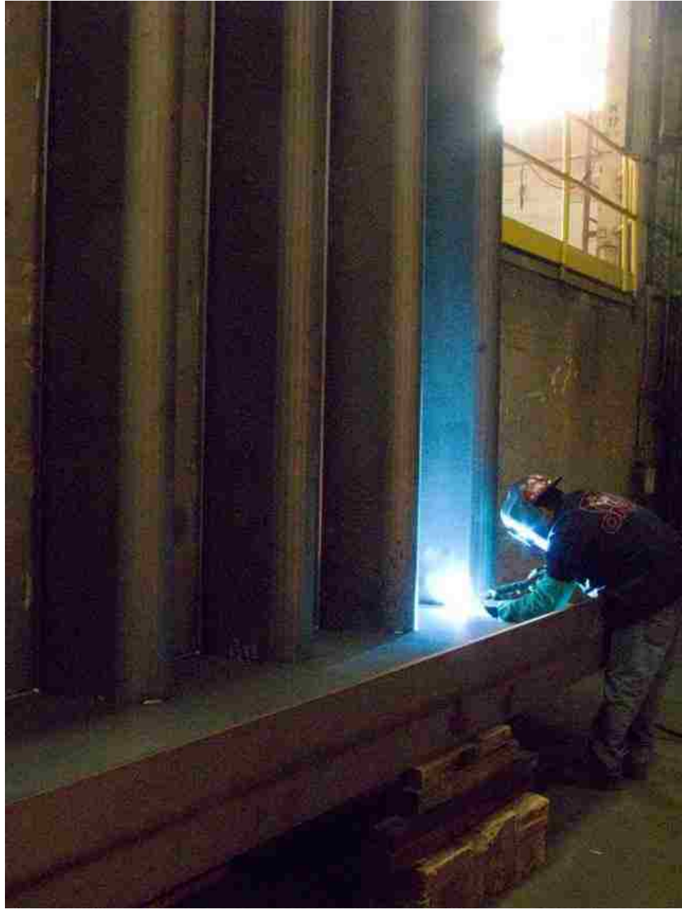
Figure 101 Rib-to-floor beam welding in 2F position
